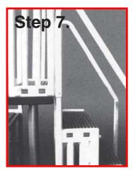
Attach the handrails, to the inside unit only, as described in step 11 of the STEP-1 instructions.
