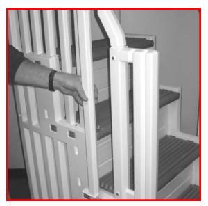
Align one of the triple pickets into the notches of the handrail at the top of the unit. Fasten the pickets in place, at the top of the pickets, using the #10 x 3/4" screws. Continue placing and fastening the double pickets and then the single picket. Repeat for the opposite handrail. Cover the ends of the screws with the protective caps.
