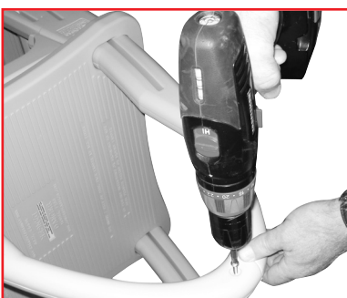
#7: Install right and left ladder bridges.
